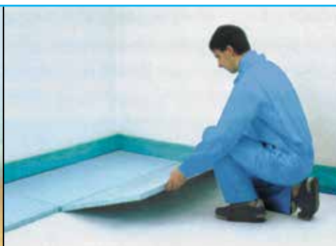
Laying of the insulating panels.
