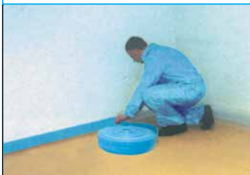
Fixing of the perimeter strip with welded PE sheet.
